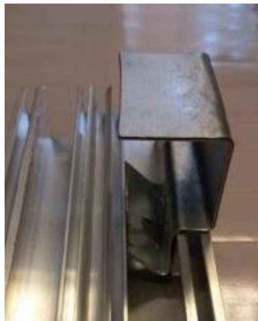
Figure 52 Bracket fitted in N80 profile
