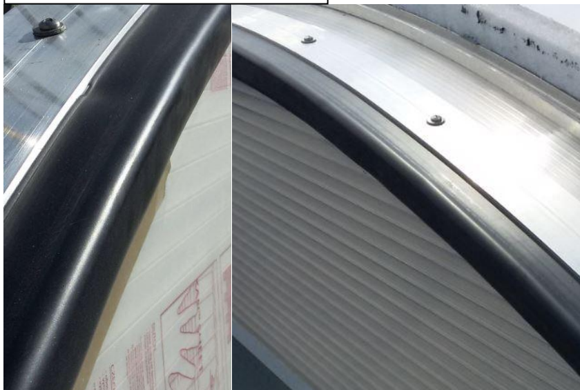
Masking gasket for tympanum panel
