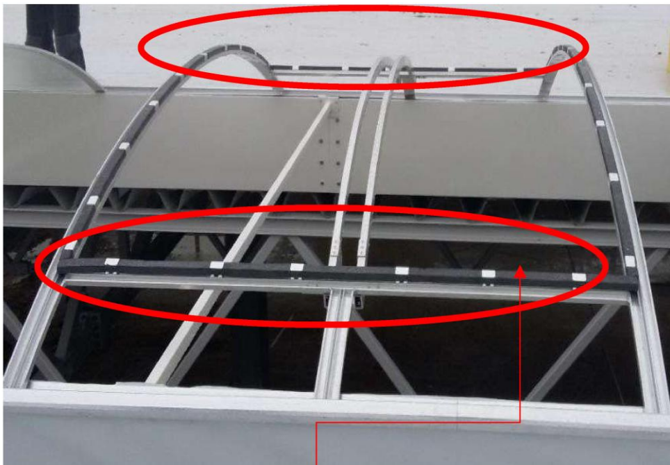
Figure 55 Layout of brackets on the vent support frame
