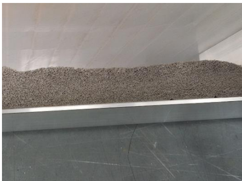
Figure 42 Expanding sealant tape right after application
